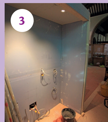
Sink/drainage area behind small partition
