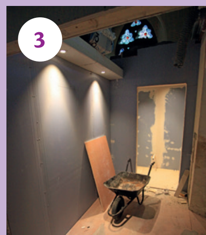
View into new lobby and smaller toilet
